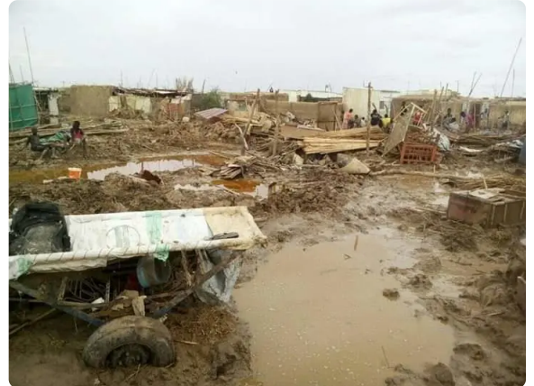
Heavy rain and flood damage in Gaboush neighbourhood, Mayo area, Khartoum
